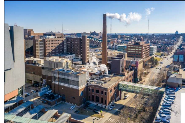
Confidential - Property of ASRC Industrial
