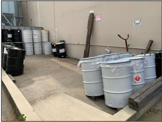
Secondary Containment / Dikes / Berms
