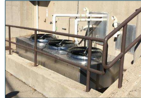
FLUID COOLER AT 911 COMMUNICATIONS
